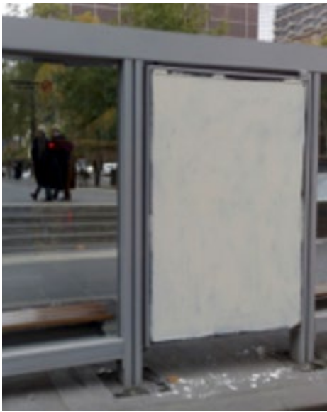
Figure 15. Tram shelter outside County Court, Melbourne. Photograph © Kyle Magee
