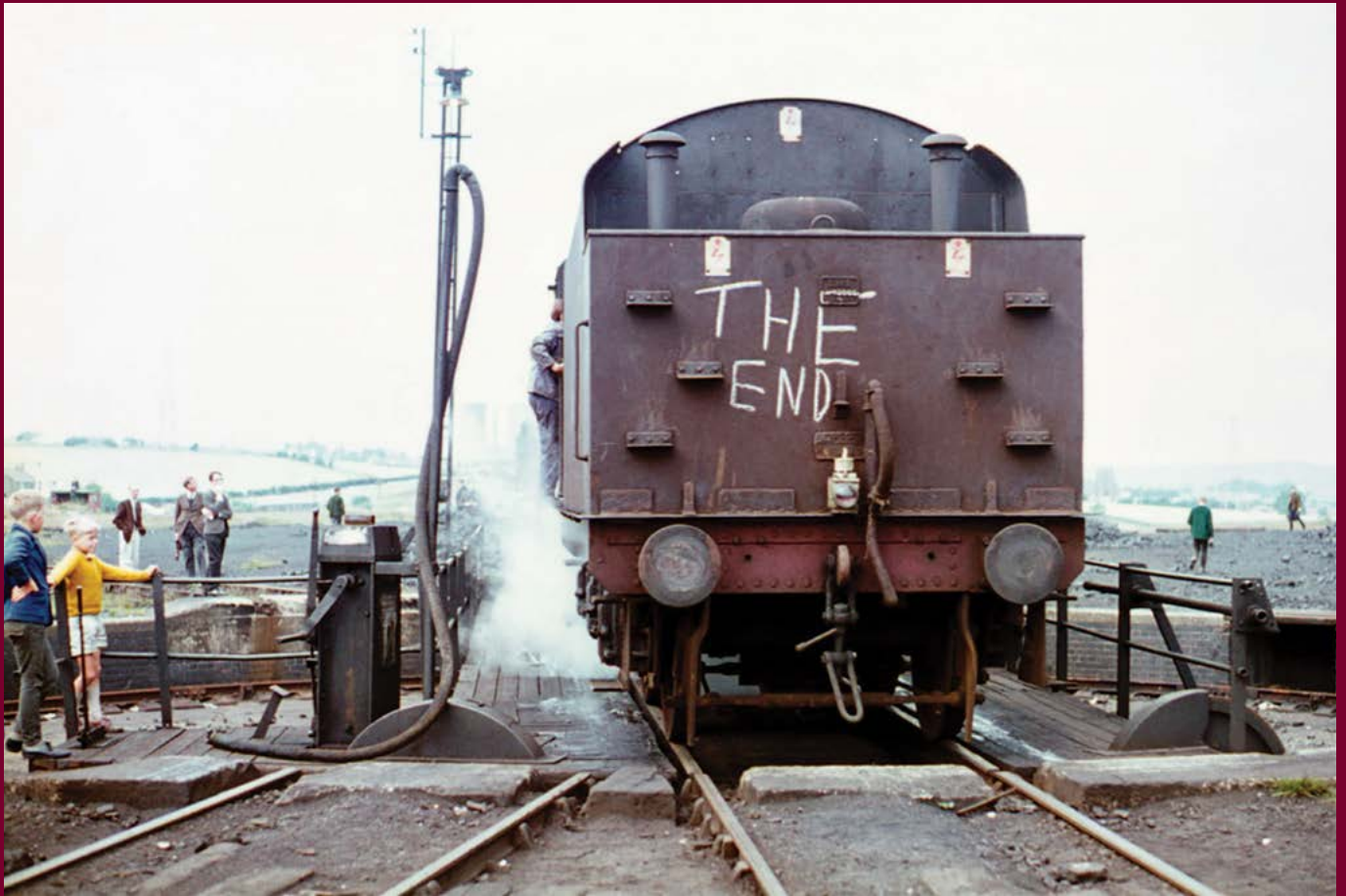
Figure 8. The End, Rose Grove, August 4, 1968. Photograph ©Martin Gemmell.
