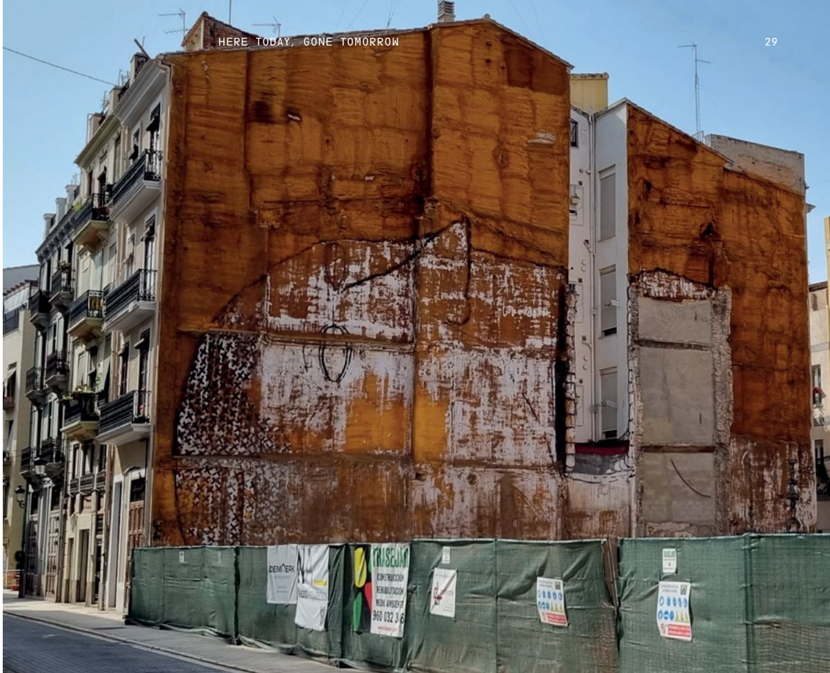
Blu. Valencia, Spain, May 2023. Twelve years after the Italian artist had painted this wall (without any scaffolding or cherry picker, just ladders and extendable painting devices), the orange-coloured spray foam coating that can often be found on the side of buildings in Spain, was clearly having the better of the once dominant white paint.
